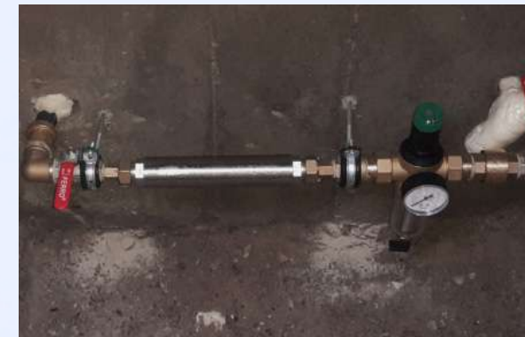
Inlet with MWD G1" PN10 in a family house
