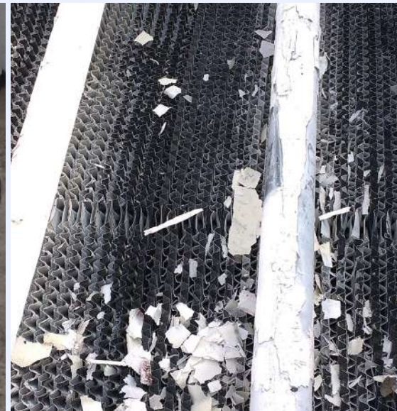
CLOGGED COOLING WATER COOLER AND CLEAN AFTER USE OF MWD INDUSTRY G2 "PN16
