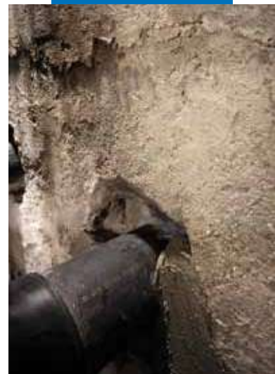
Uzavretie Mapeproof Swell cementovou maltou Mapegrout T40
