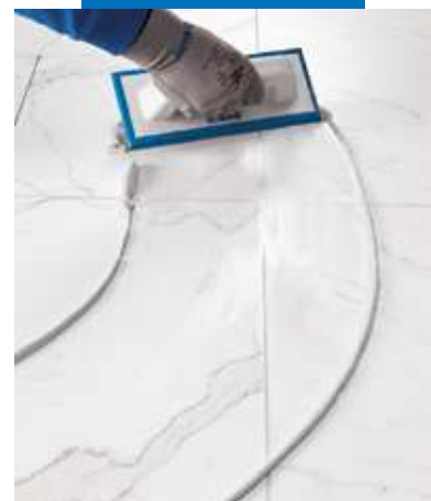
Spreading Ultracolor Plus on marble-effect porcelain floor tiles with a rubber float
