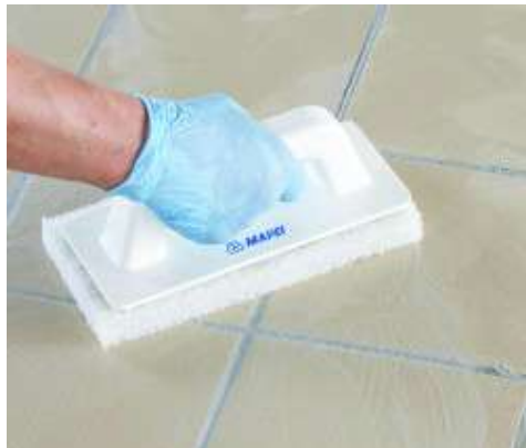
Cleaning joints with Scotch-Brite®
