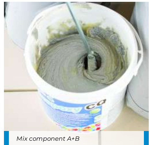
Pour the hardener (component B) in the container of component A
