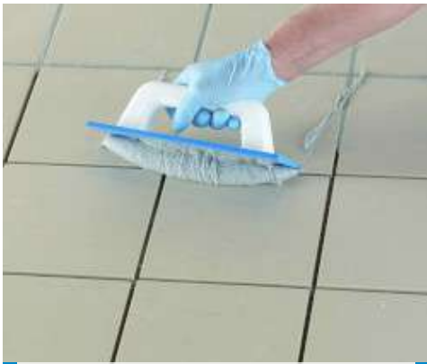
Application of Kerapoxy CQ with Mapei rubber trowel
